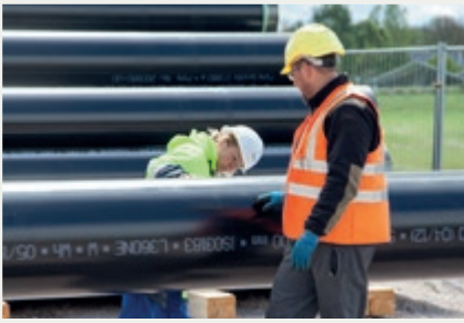
Each pipe consignment from over 760 truckloads is closely inspected.
