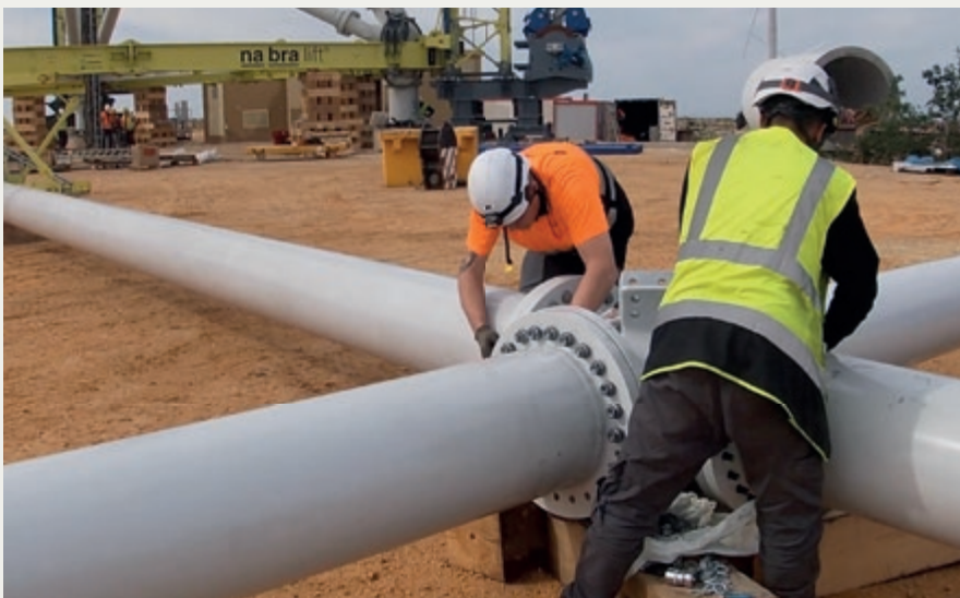
Above: The HFI-welded tubes manufactured in Hamm and Siegen were further processed in Spain before being shipped to Morocco.
