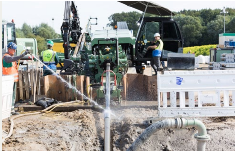
Bottom left and above: At a total of 14 points, the up to 1.9 km long pipe strings were trenchlessly laid by HDD with minimal impact on the natural environment.
