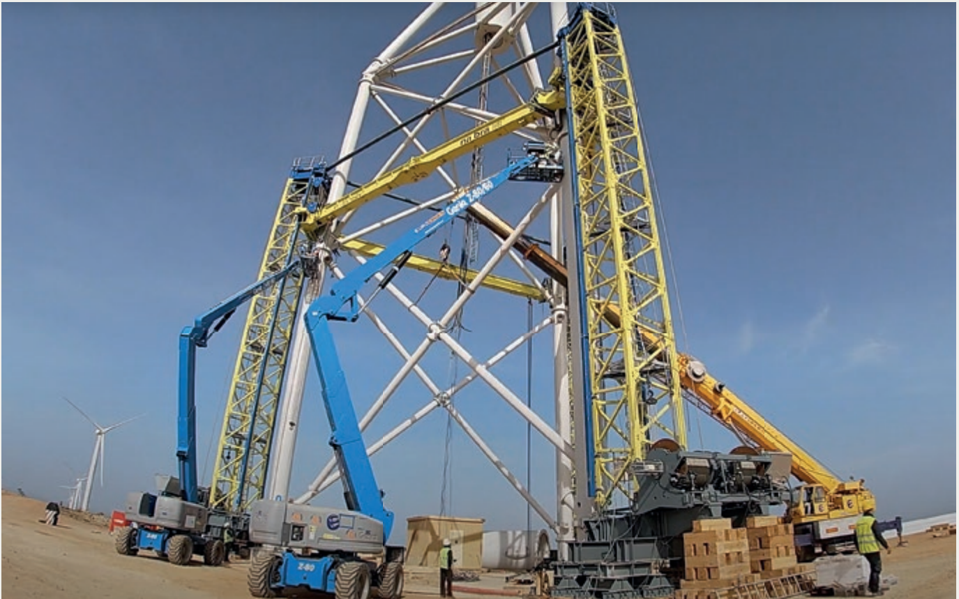
The SES in action. The second tower unit with the steel tubes supplied by Mannesmann Line Pipe is assembled and connected to the unit above.
