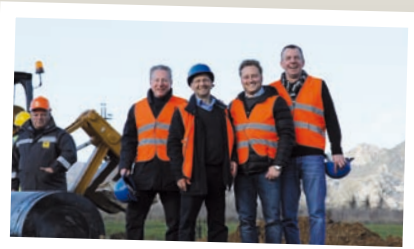
2. Italy From left to right: Andrea Jachetti (Sinter-tec srl), Vincent Bertolone, Domenico Tinaro, Società Gas Italia (SGI), and Michael Kosfeld, on the construction site of a high-pressure gas pipeline
