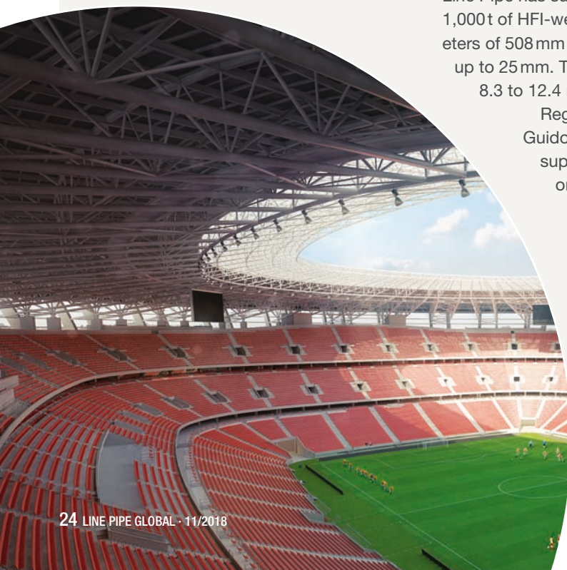
Left: The HFI-welded tubes from Mannesmann Line Pipe are key structural elements of the new stadium's roof structure. Image: ©www.mnsk.hu
