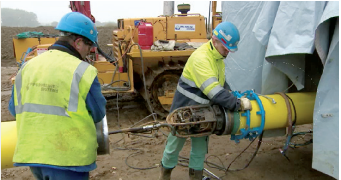
Aligning steel pipes on the construction site
