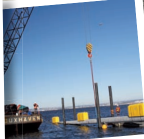
Offshore pipe-laying operations
