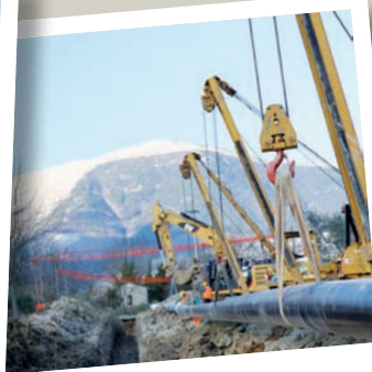
The pipe-laying contract was awarded by Società Gas Italia (SGI)
